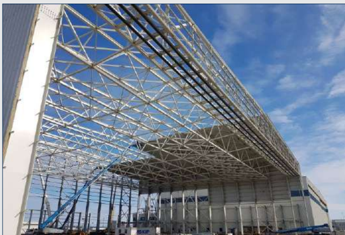
Hangar Aviativ | 14.000 mp | Reykjavik, Islanda • 1.350 tone structuri metalice
